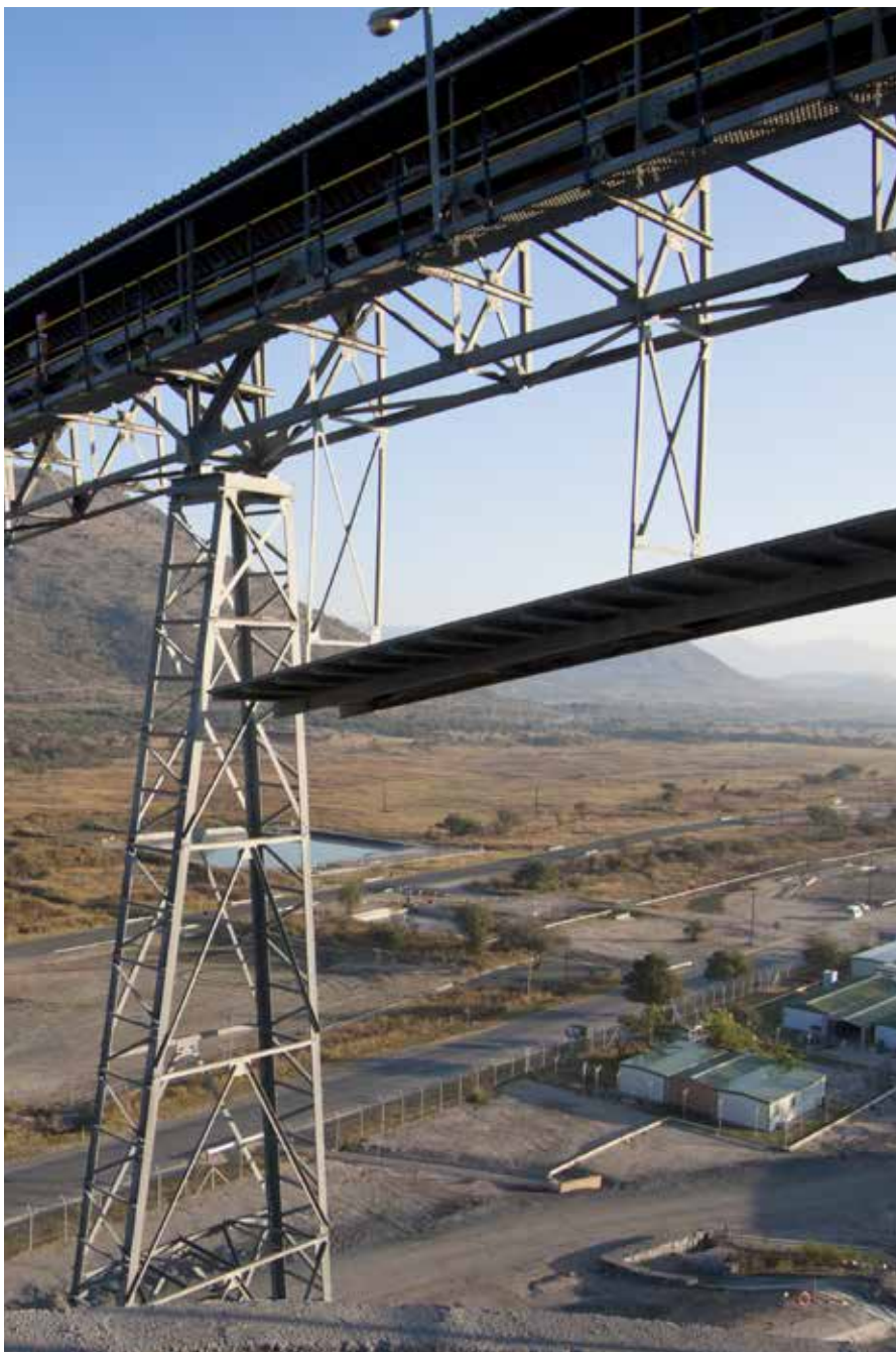
Overland conveyor belt, Two Rivers.
