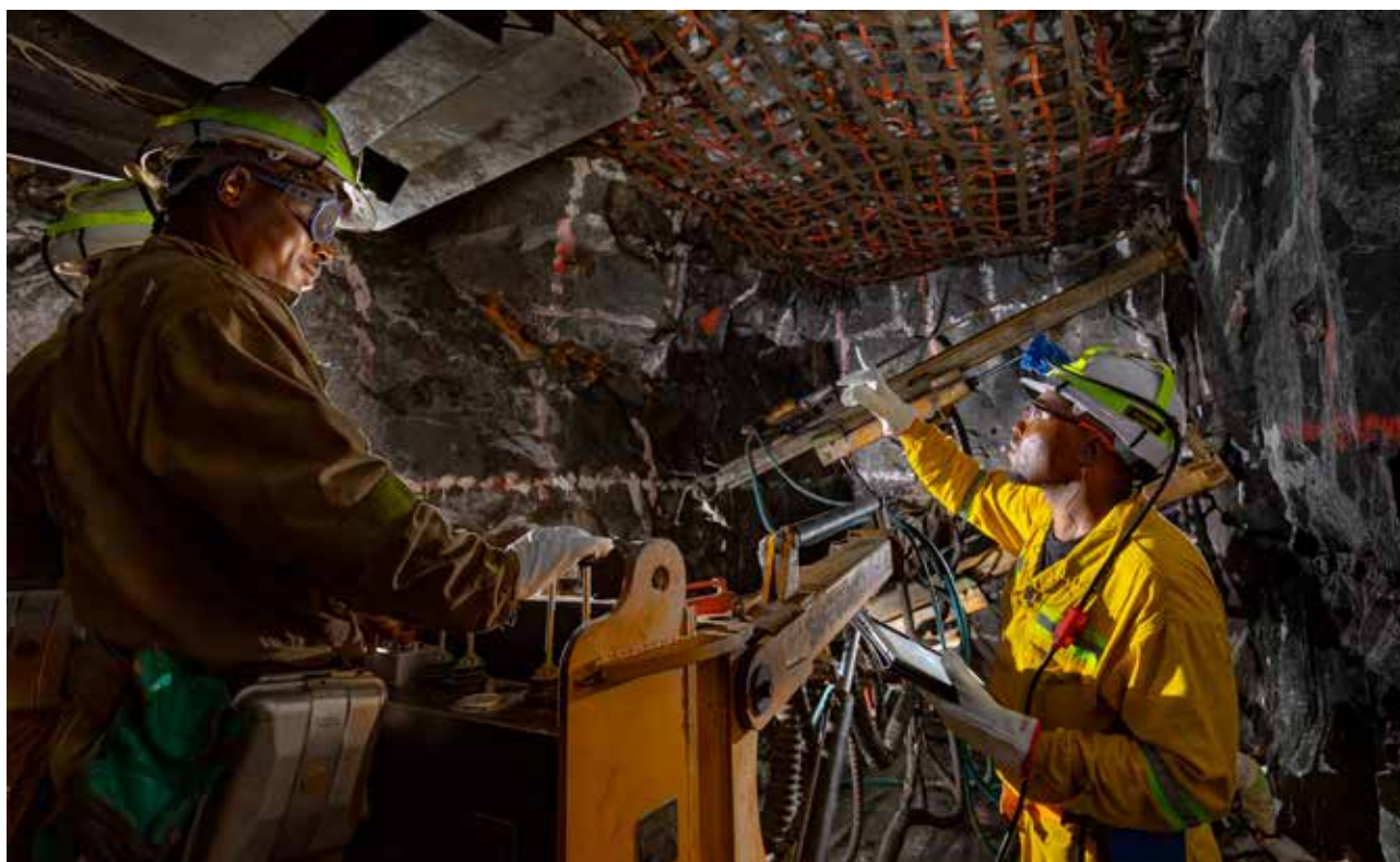
Development rig at North shaft Phase III hybrid mining section
