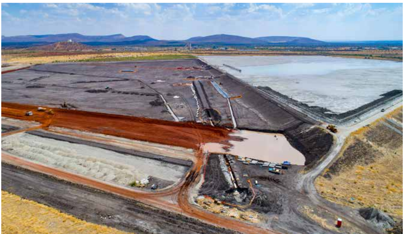
The expansion of the Maseve tailings storage facility under way
