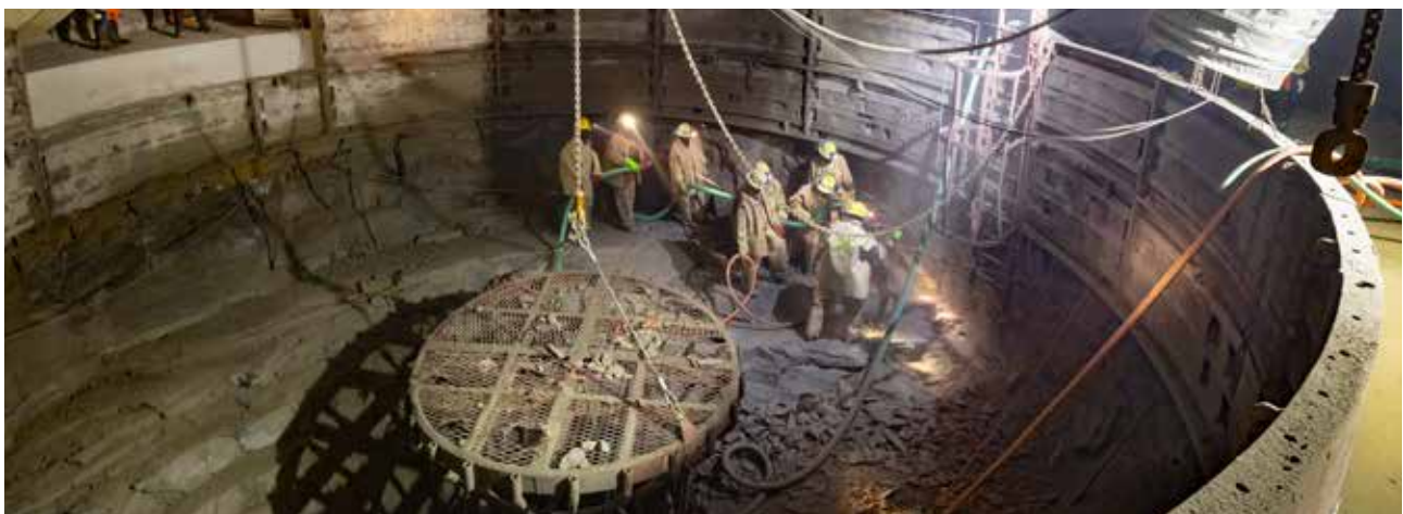
Styldrift Settler No 2 collar construction
