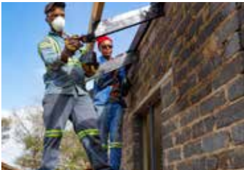
Construction work on a community house
