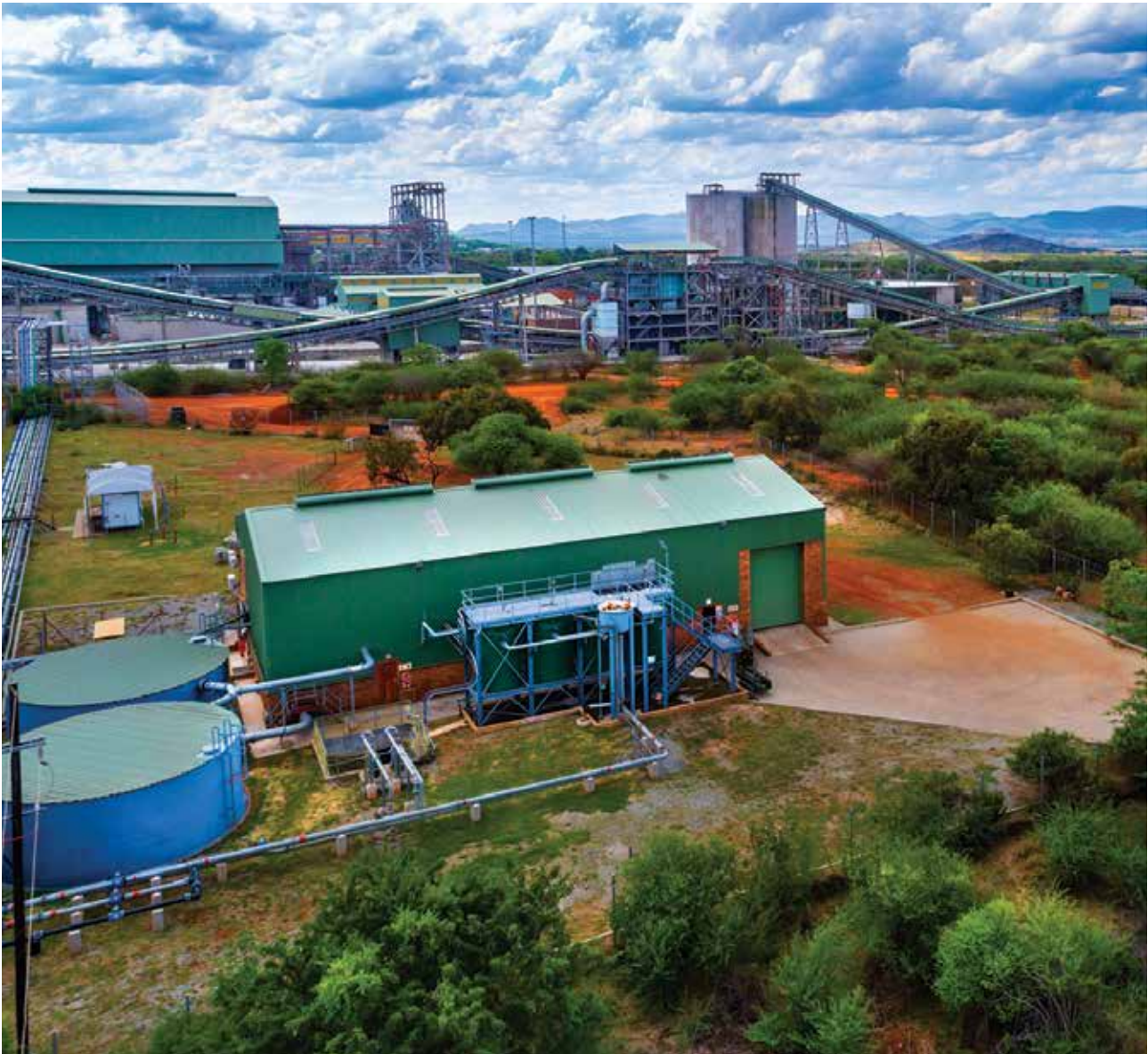
BRPM with the water treatment plant in the foreground
