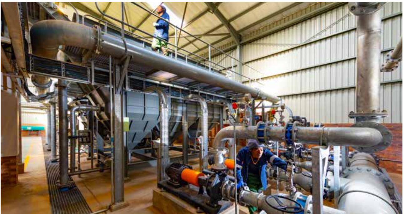
The water treatment plant at BRPM
