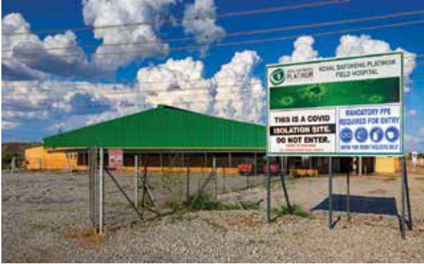
The 200-bed field hospital RBPlat established to ensure medical facilities would be available to our employees and communities during Covid-19
