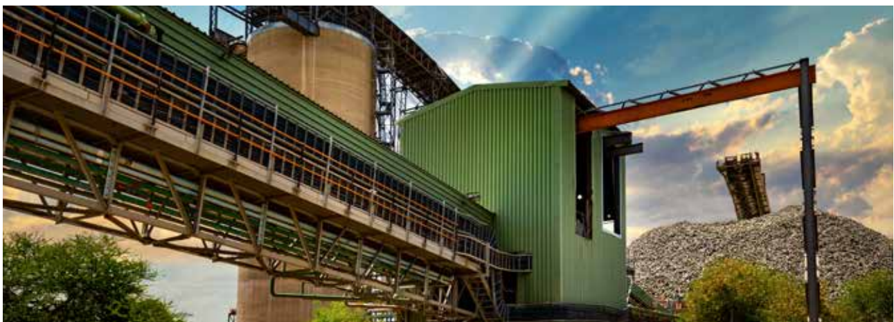
The silo at the BRPM concentrator
