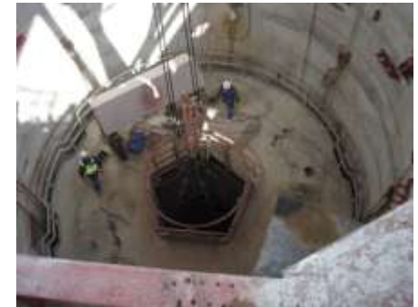
Sinking activities commencement
