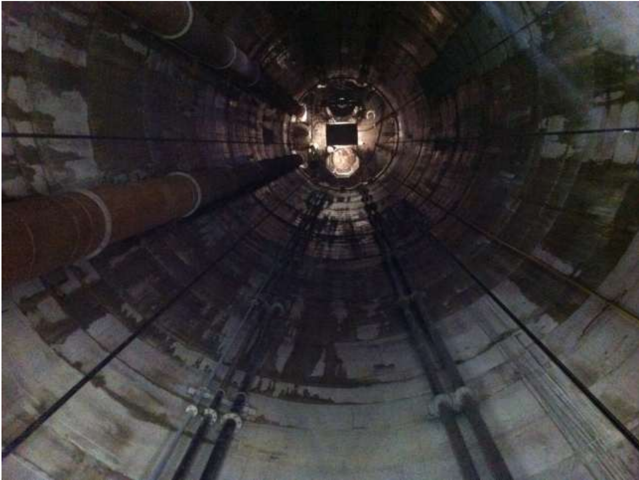
Sinking in progress
