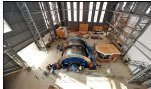
Major equipment installation
