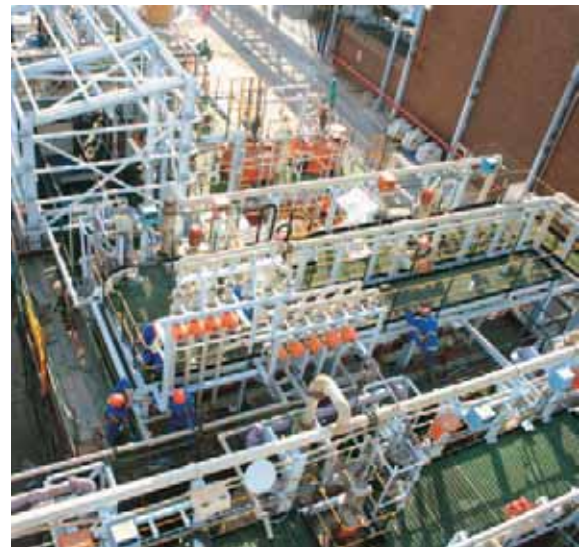
Construction in the EPMR tank farm area, Refineries.
