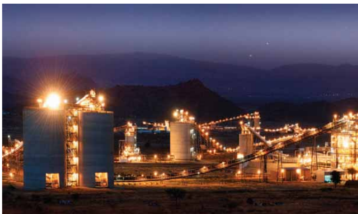
The Marula Platinum mine at night.
