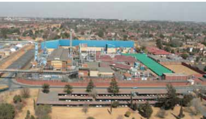
An aerial view of the Precious Metals Refinery, which clearly illustrates the close proximity of the plant to the Springs community.
