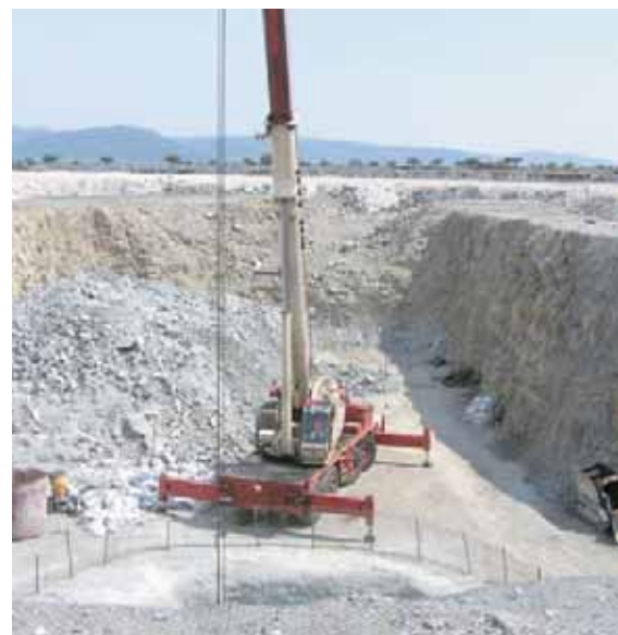
Sinking of the new No. 20 Shaft at our Rustenburg operations.
