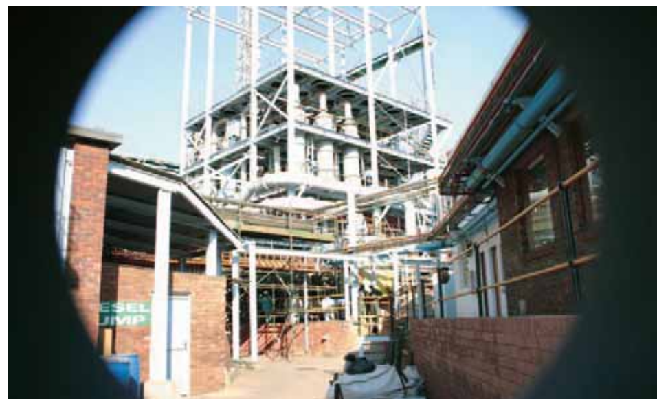
The primary air scrubbing system at the Precious Metals Refinery, prior to emission into the atmosphere.
