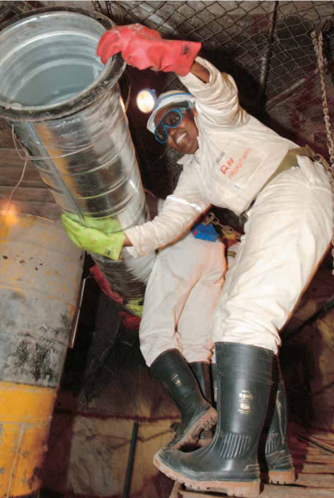
Employees place a ventilation pipe underground, wearing comprehensive personal protection equipment.
