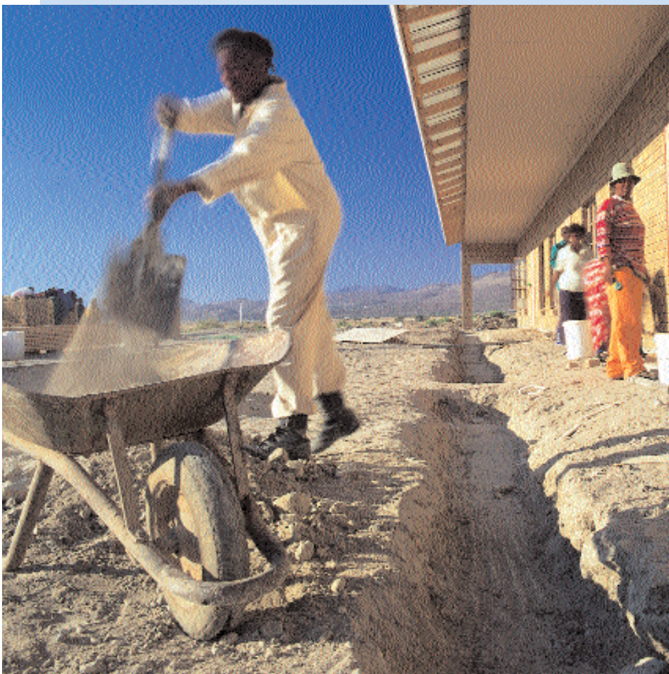
Above and left: Extensive consultation with the governing body of the local school resulted in the construction and equipping of a new school
