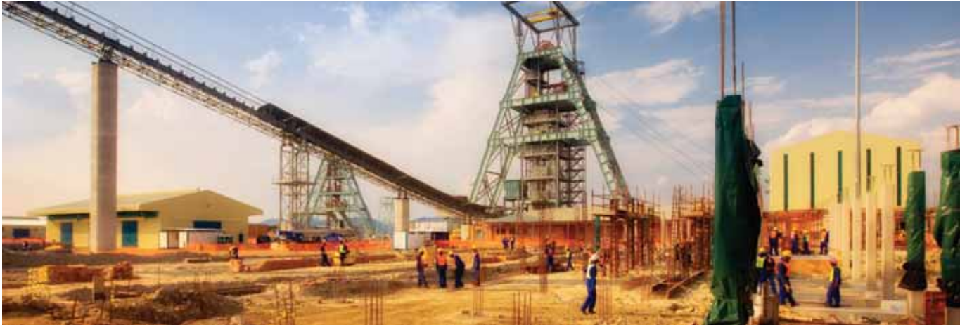
Shaft construction at Impala
