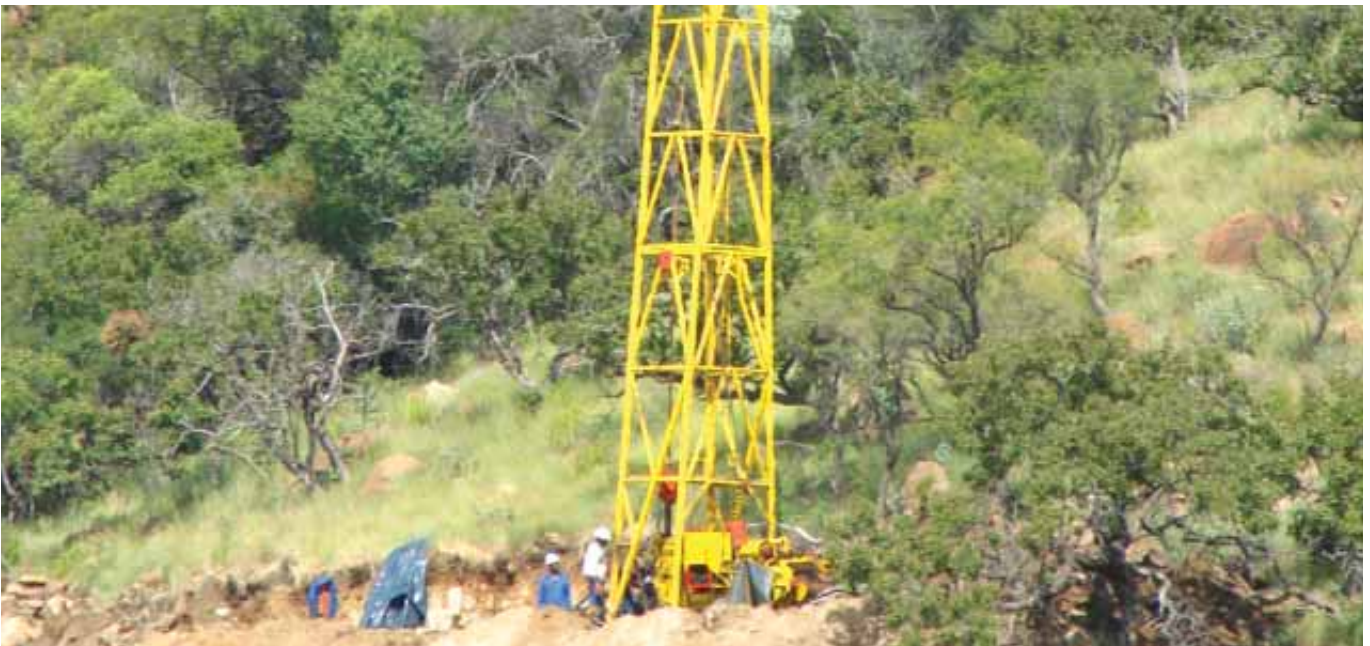
Drilling in progress on Tamboti project
