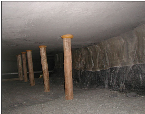
View down the panel towards the drive
