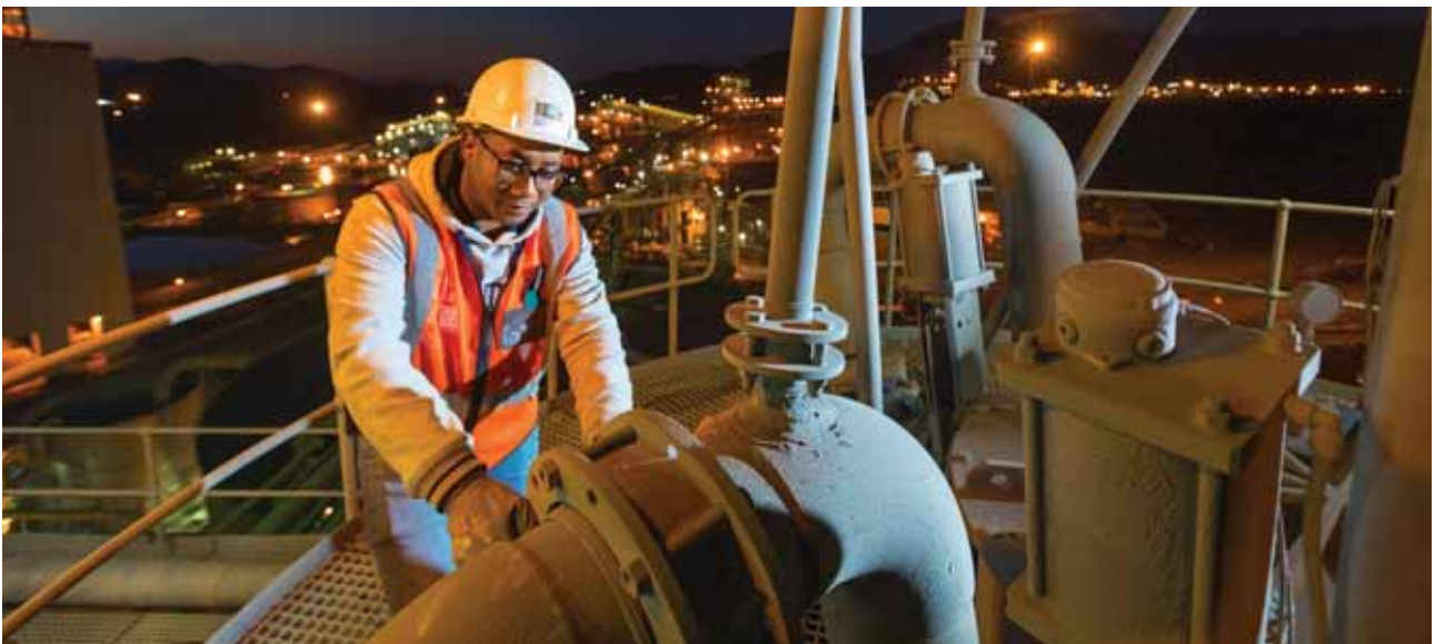
PLANT MAINTENANCE, TWO RIVERS
