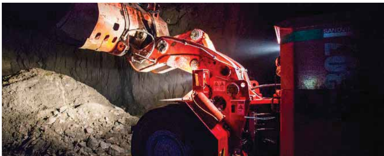
ORE MUCKING UNDERGROUND, MARULA
