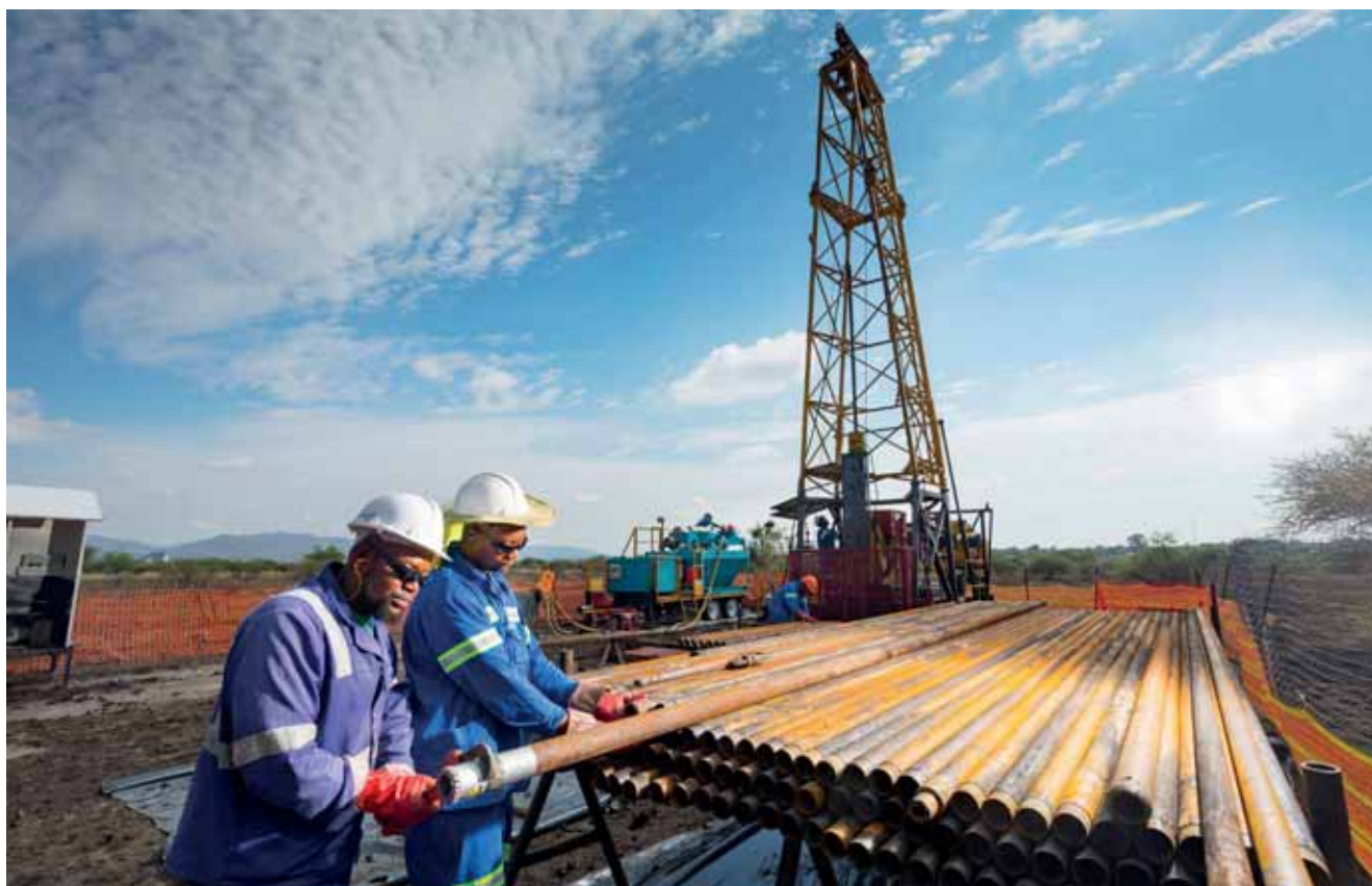
Exploration drilling operation, diamond drill bit replacement, Styldrift I
