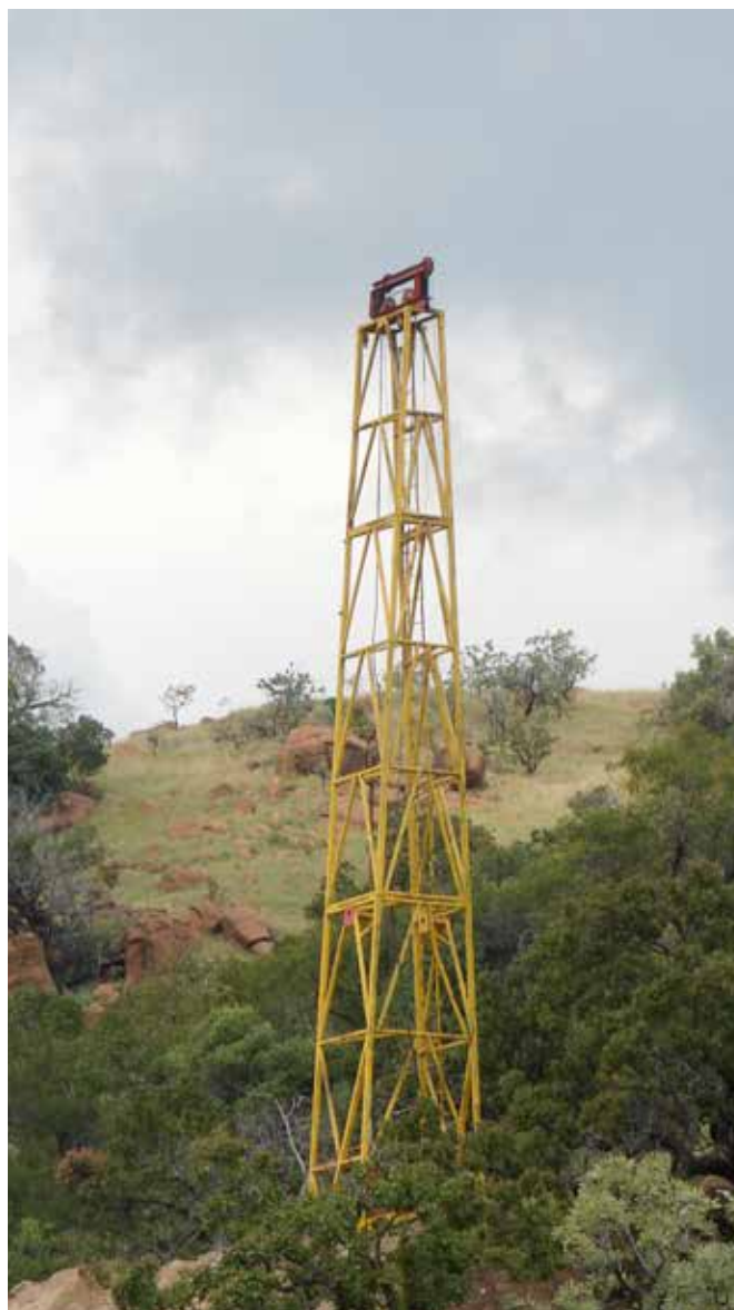
Tamboti drilling tower – Kalkfontein
